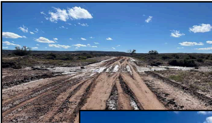
* Flooded wash crossing 1. Route N-9003 35.5154, -109.8491
